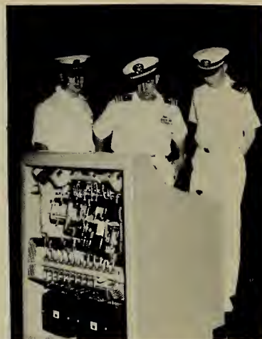
Officers and Midshipman examine "Bailey Board" which controls combustion and feed water
