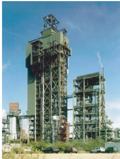
Fig. 8.1. HTW plant in Berrenrath, Germany
